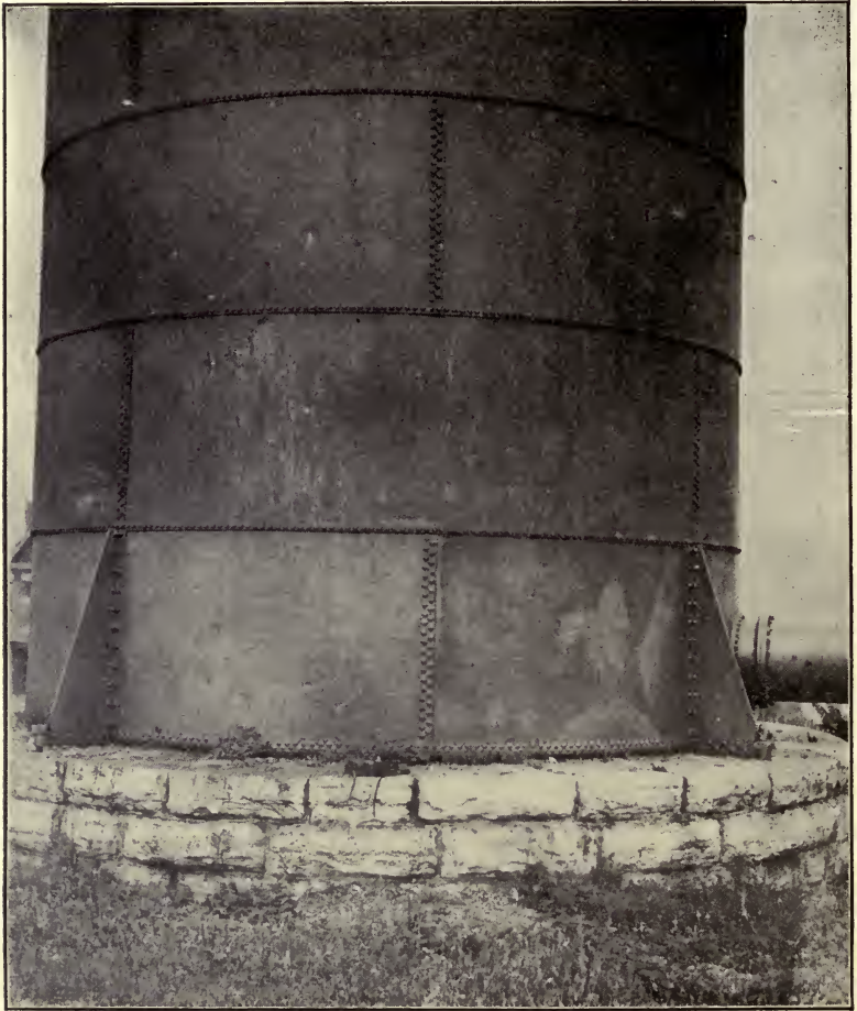
FIG. 9b.—Anchorage for 24 ft. \times 70 ft. Stand-pipe.
